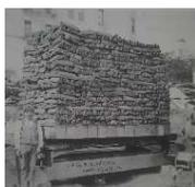
McKim’s **design specified load capacity of 500#/sq.ft.**, so on **April 20, 1889** Guastavino **built a small vault section to test the loading** of 12,200#/22sq.ft. (550#/sq.ft.). **May 9, 1889 drawings were altered for Guastavino system** and on **May 14, 1889 given the contract to substitute tile vaults for iron beams**. Put out to bid, with **Guastavino the only bid, since the system was patented** (1885). From the commission, he founded the **Guastavino Fireproof Construction Company**.
