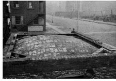
After winning the bid for constructing the vaults for the **Boston Public Library** in **May of 1889**, Guastavino was invited to **lecture on the Theory and History of Cohesive Construction** (made of adhesive cement mortar, as opposed to Gravity Construction with Stone) **applied to the Timbrel Vault** (made of bricks on end), delivered to the Society of Arts at MIT on **October 24th 1889**, he noted:
