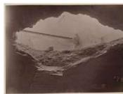
**Hole created through an arch** of a Guastavino vault, during the construction of the Boston Public Library, when a **2 ton stone fell** from work above (1889). Both the **arch and vault around the hole remained intact**, did not fall, **proving the strength** of the structural tile system.
