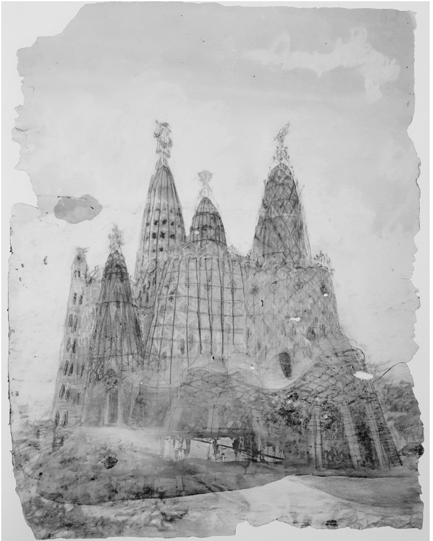
Colònia Güell Church, painted in gouache by Antoni Gaudí over inverted photograph, 1910. Note the inclined columns with strings visible from the underlaid photograph of the stereo-static model.
