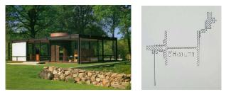
Ground was broken on March 20, 1948 and construction began. Full-sized drawings of the steel details for mullions, cornice, corner posts, and door jambs, with specifications for 18 ft. sheets of glass were sent to New York for fabrication.
