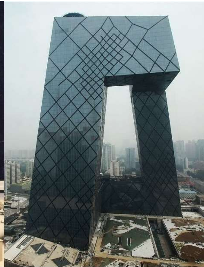
CCTV Headquarters (Koolhaas - 2002)
